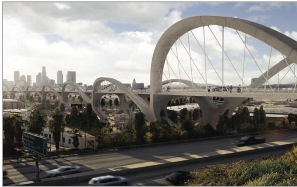
Los Angeles, CA – Sixth Street Viaduct
