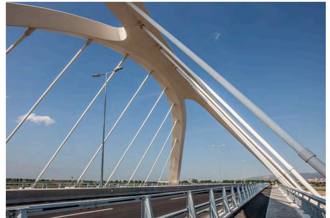
NELSON MANDELA BRIDGE, BARCELONA, SPAIN
