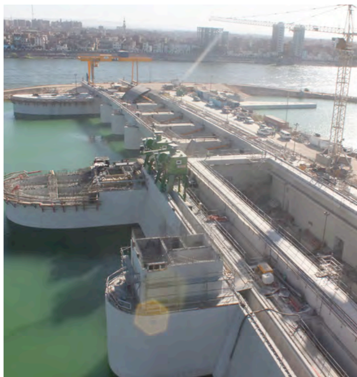
ASSIUT BARRAGE AND HYDRO-POWER PLANT, EGYPT
