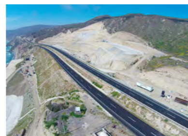
Infrastructure: Restitution of Embankment in Tijuana-Ensenada Highway at KM 93 Ensenada, Mexico
