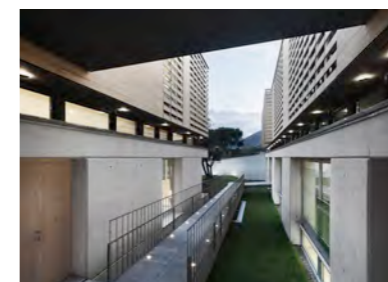
SPECIAL PRIZE Sustainable Building: Oak House School Barcelona, Spain
